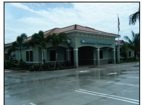
Seacoast National Bank built with Redi-Tilt™ in Port St. Lucie, FL
