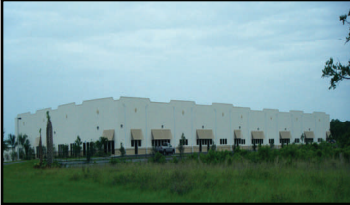
LTC Parkway Distribution Center in St. Lucie County, FL; One Of Two 70,000 Dock-Height Buildings Under Construction
