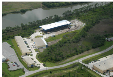
Poma Construction Corp./Redi-Tilt™ Headquarters in Palm City, Florida
