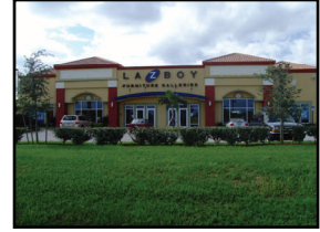
Constructed with Redi-Tilt™ Precast Wall Panels, La-Z-Boy anchors this retail center on US 1 in Jensen Beach, FL
